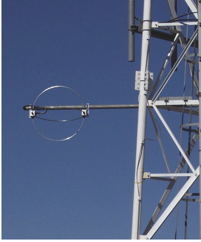
Figure 3.3: The beacon antenna mounted on the communication tower at Coihueco [33]. It is an antenna of type SALLA with a diameter of 75 cm, continuously transmitting sine waves into the field of AERA.
