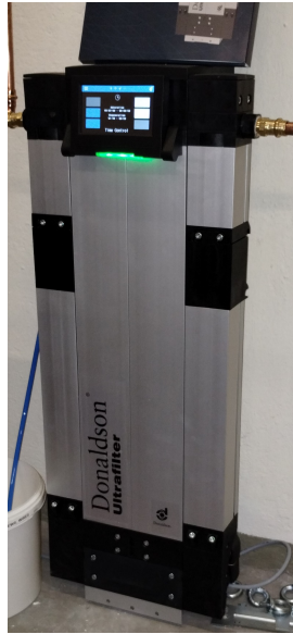
Figure 4.5: Donaldson Ultrafilter air dryer installed in the basement of University of Siegen Emmy-Noether-Campus Building A.
